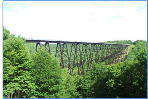
The Kinzua Viaduct
