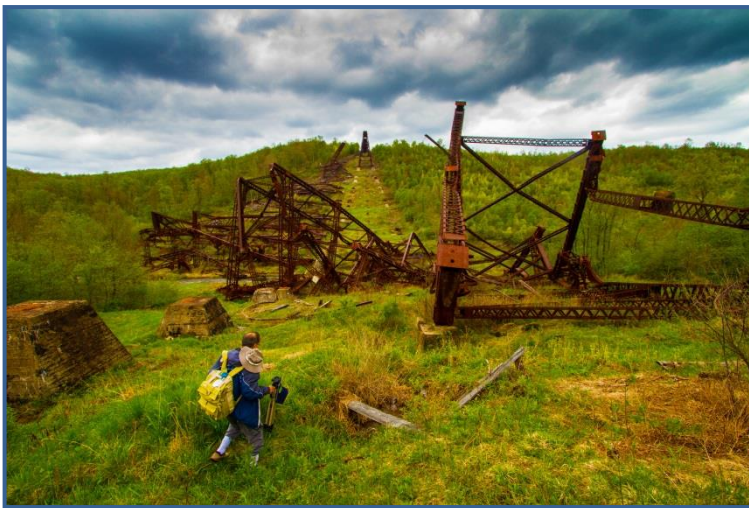
This is the view underneath of what remains of the bridge.
